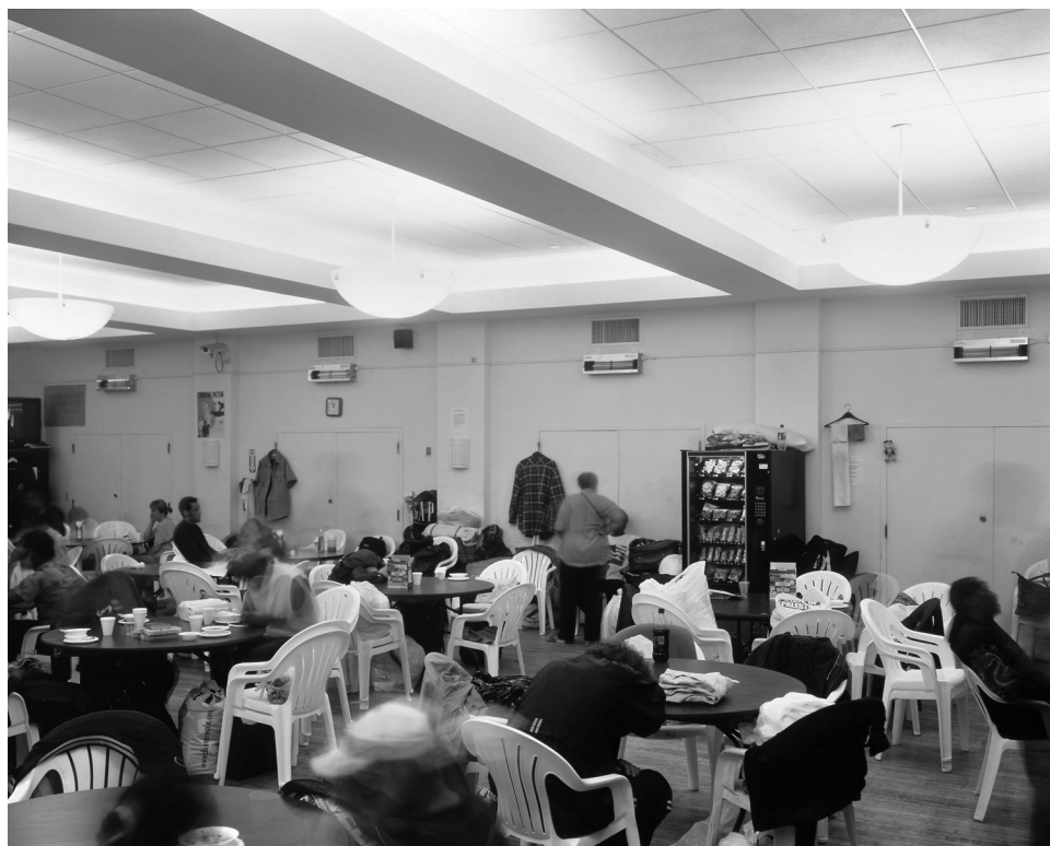
Tuberculosis Ultraviolet Shelter Study New York City shelter in a church basement. Note the ultraviolet germicidal irradiation fixtures located on the upper wall, directly below the vents. Photo: ©Randall Perry Photography.
