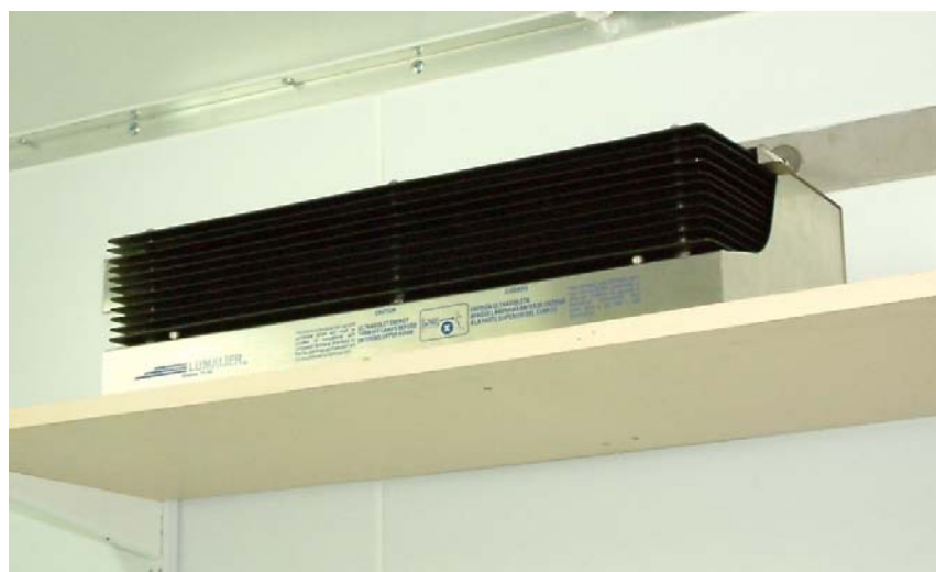
Plate 5. Wall mounted open field UV device (Lumalier, Memphis, USA)
